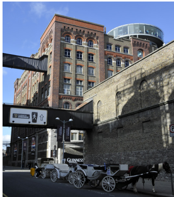
Guinness Storehouse in Dublin
